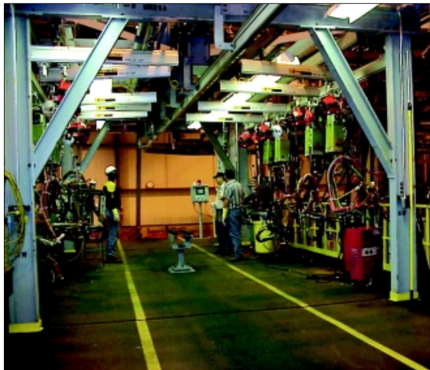
IR Zimmerman rail system application shown in a manufacturing facility.
